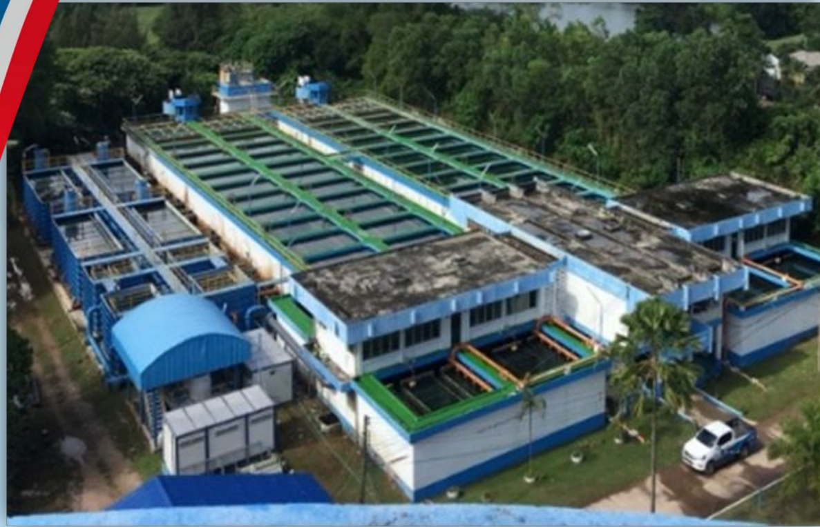
Bang Wad Water Treatment Plant
