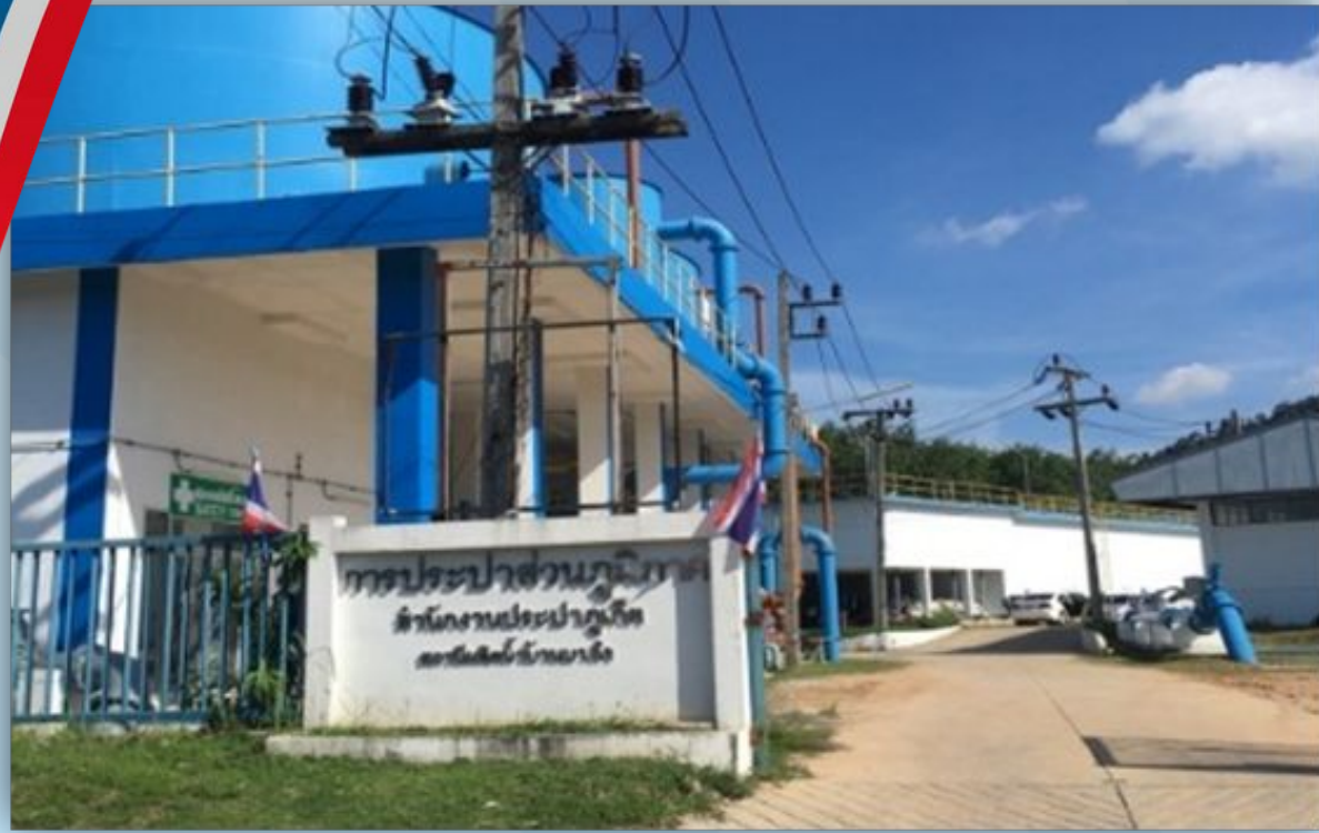
Bang Jo Water Treatment Plant
